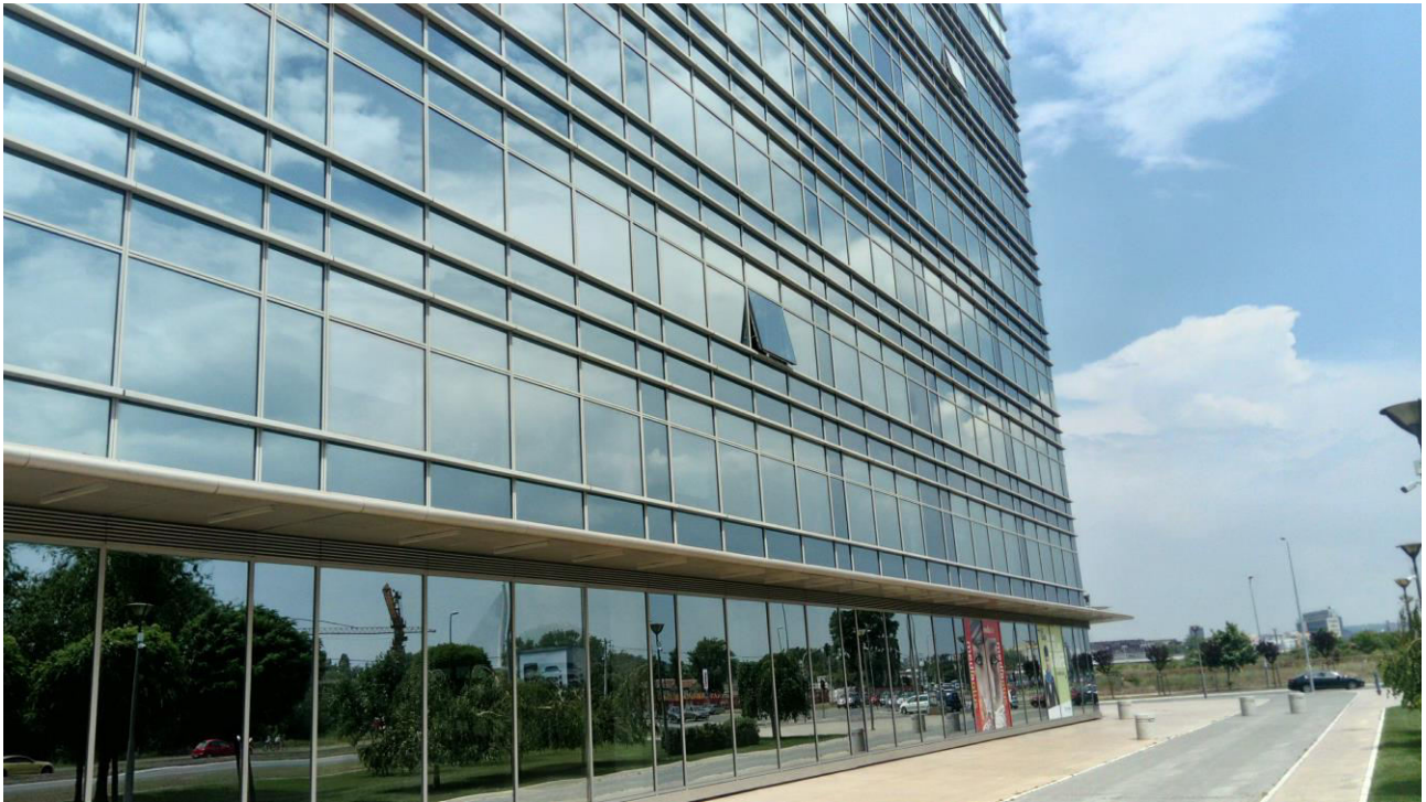
Figure 1. An example of an air-conditioned building with windows that can be opened.
